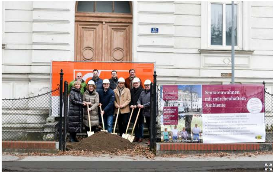
Der Spatenstich in Melk (c) Silver Living
